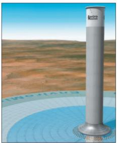
RENDERING PROVIDED BY ENVIROMISSION INC. Phoenix-based EnviroMission Inc., a subsidiary of an Australian company, is looking to bring a form of solar technology to Arizona that will turn hot air into energy without using water.
